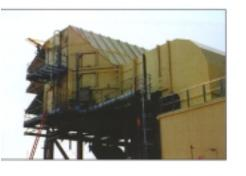
The AMER-Kool III unit has been designed to provide maximum performance with minimum pressure loss. Air to water contact is achieved in a fluted media. The large fluted openings are positioned to create the maximum evaporating interface between the air and wetted surfaces. This permits the AMER-Kool III to operate with minimal pressure loss and negligible water carry-over.
